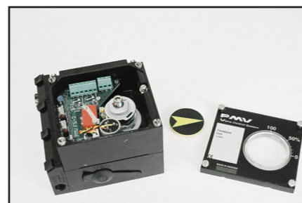
Install indicator and cover
